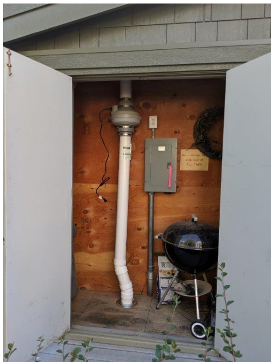
Placement of suction fan and discharge pipe in the owner electrical closet.
