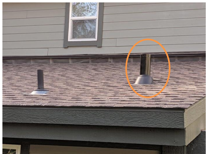
Roof penetration above Electrical Closet
